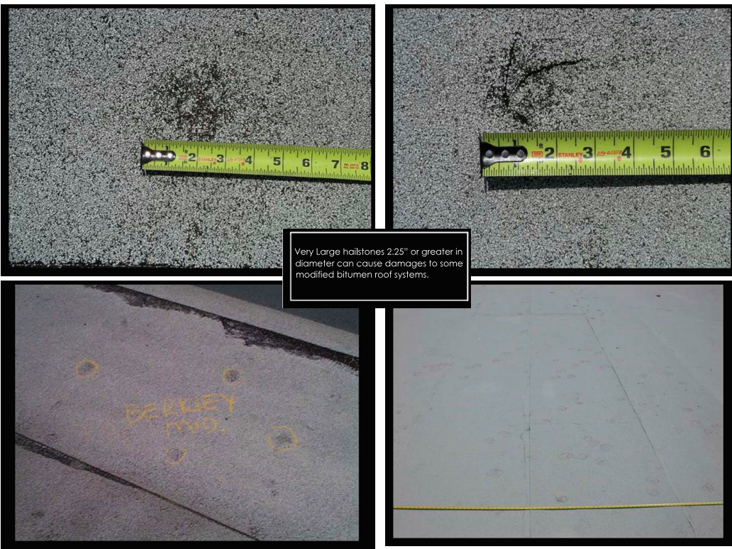
Frequent and very large hailstones impact marks 2.25" or greater in diameter can be seen in these photos.
